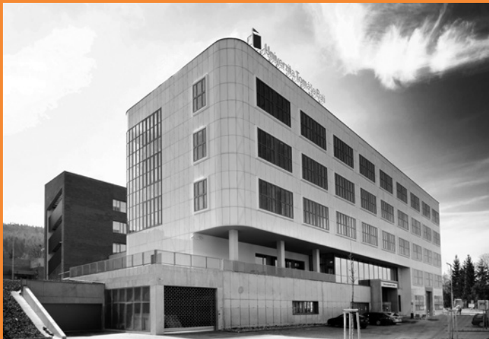
Late in the year, the construction of a top-level scientific and research unit - the Centre of Polymer Systems - was completed.
